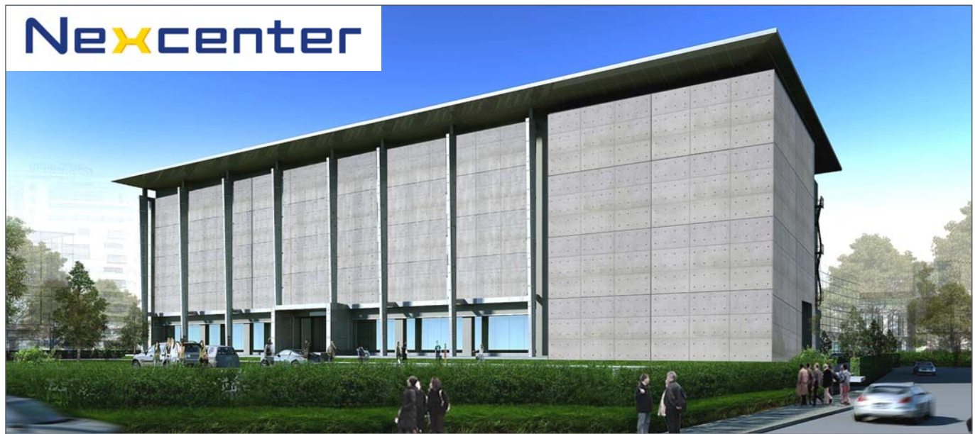
Thailand Bangkok 2 Data Center
